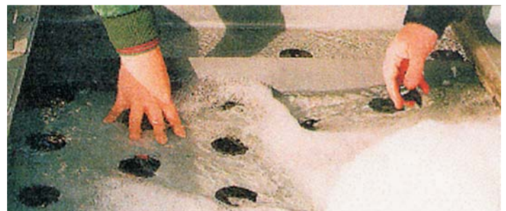
Problems solved & pans protected with CHEMCLAD SC.
