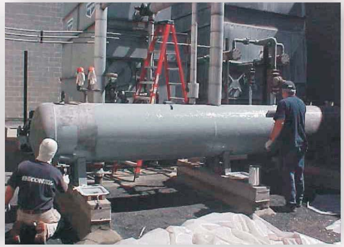
First coat of CHEMCLAD SC being roller-applied to tank and support surfaces.
