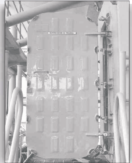
Same door protected with CHEMCLAD SC
