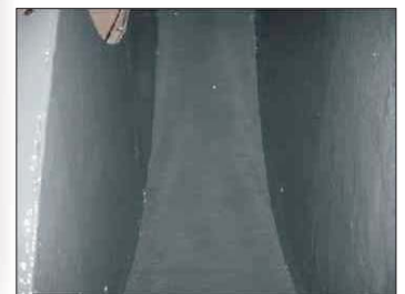
Two coats of CHEMCLAD XC were applied to all interior surfaces and flanges.
