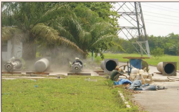
All pump sections were grit blasted.
