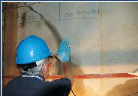
A variety of repair procedures - including crack injection - were tried but failed almost immediately.
