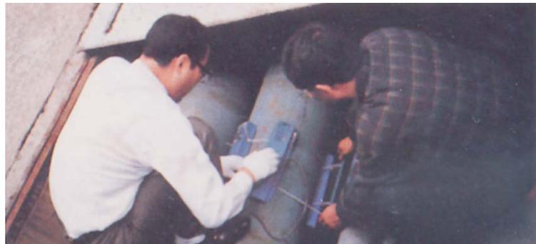
Four pair of ENEFLOW 5000 Fluid Dynamic Power Cells being installed on one of the main ash slurry lines.
