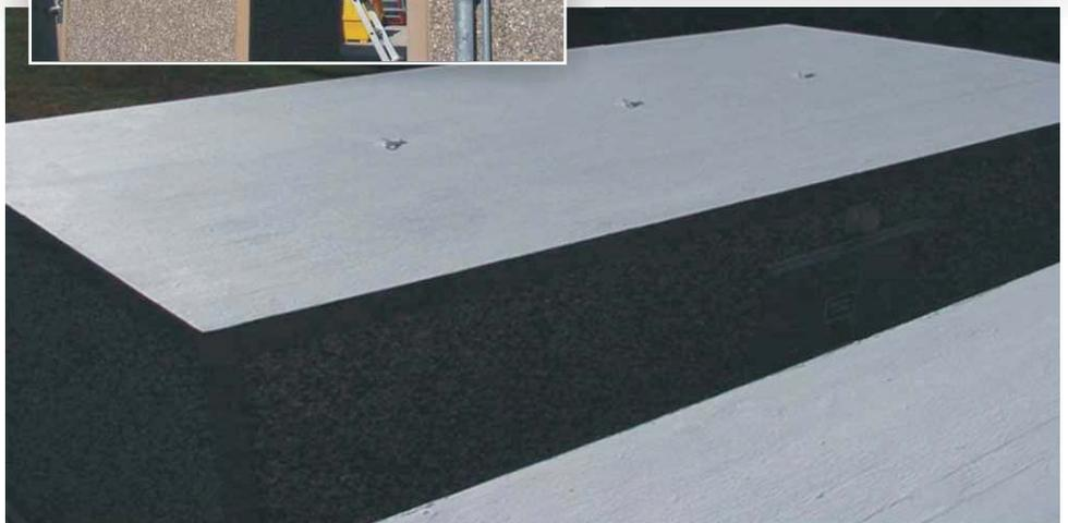
This weather station, located in the Mid Atlantic Region, had serious leaking problems through the concrete roofs which were affecting the sensitive electronic weather monitoring equipment located in these pre-fabricated buildings. The existing roof coating had failed and water was
