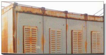
These electrical cabinets at a sewage treatment plant in Tennessee were severely corroded and needed immediate remedial work. The plant engineers wanted a surface tolerant, corrosion protection coating system with minimal V.O.C. issues.
