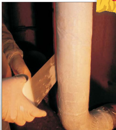
Fiberglass reinforcement tape over 1st
