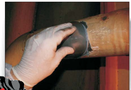
Patch applied to hole
