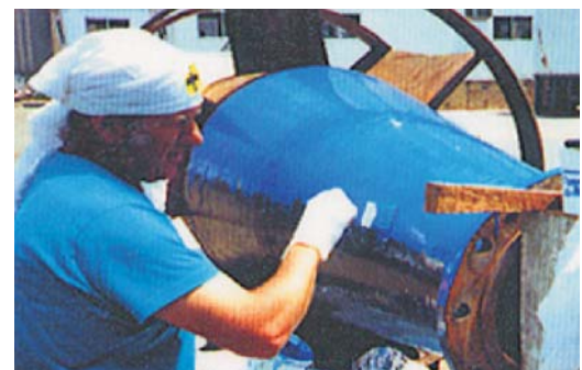
Applying CL+ to one of the diffuser components.
