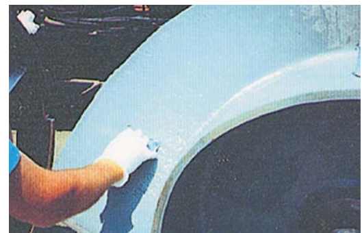
Rebuilding with CeramAlloy CP+
