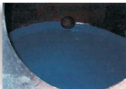
Water box repaired & coated
