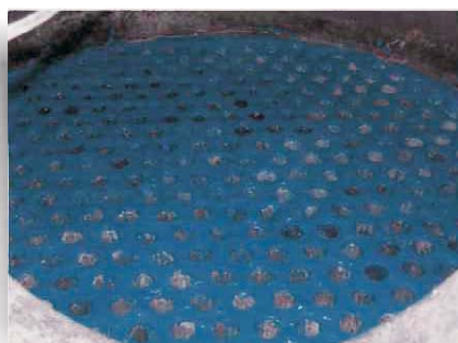
Tube sheet repaired & protected
