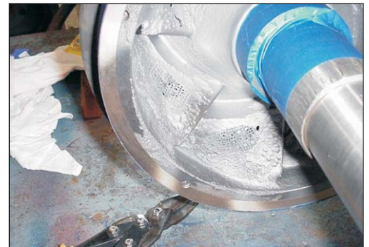
Reinforcing 'mesh' and DurAlloy applied over holes
