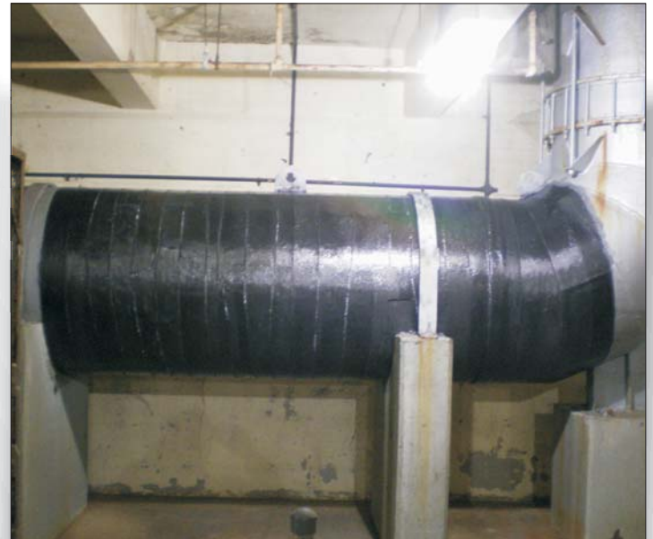
Completed DuraWrap System.
