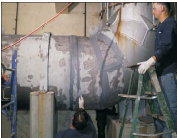
After grit blasting, leaks repaired with DurAlloy.
