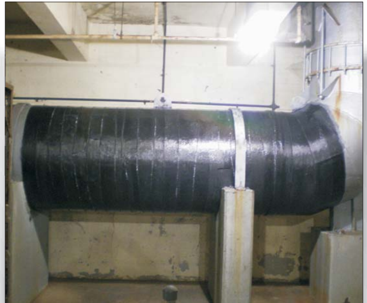
Completed DuraWrap System.
