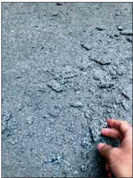
All the loose flooring material is removed
