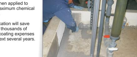
Their local ENECON Field Engineer recommended using **ENECLAD** SuperBond which is a surface tolerant primer with an extended overcoating window, followed by CHEMCLAD XC for maximum chemical protection.
