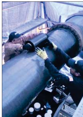
Carbon fiber pipe wrap
