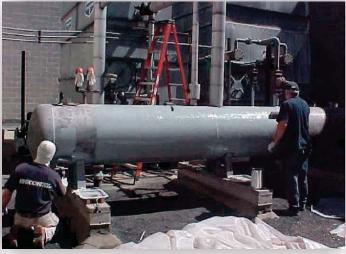
Badly rusted pressure tank and support legs. Project called for grit blasting tank and supports, then treating tank and support surfaces. with CHEMCLAD SC (2 coats).
