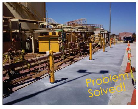
The maintenance engineers at this Laterite Nickel Mine in Western Australia had a very severe corrosion problem in this concrete loading bay. Trucks load and unload chemicals in this area 7 days a week.
