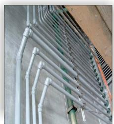
This new class of ship (twin hull, high speed catamaran) had been experiencing surface (Chief Engineer) corrosion on the hydraulic piping in the aft of the ship from salt water spray. Excess rust and staining were a result.
