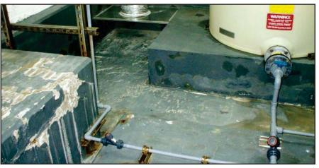
A Seattle area pump station treats water on site with 12% sodium hypochlorite. This is a high concentration to keep the system clear of bacteria and other microorganisms throughout the long pumping distances.
