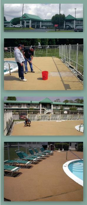
ENECON developed DuraFill for use as both a cost effective, bulk-fill material and for "broadcast" flooring applications. It has gone through well over a year of very successful field application trials.
