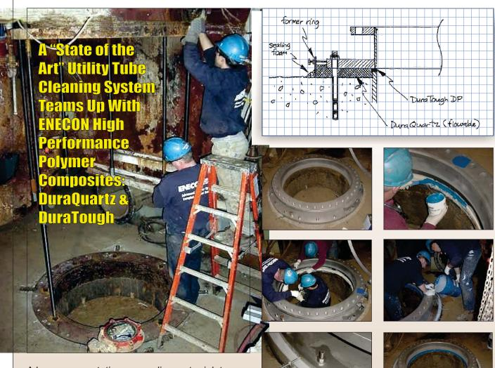
A large power station on Long Island, New York, opted to install a highly specialized tube cleaning system manufactured in Germany to keep its main condensers running at peak efficiency. However, the limited space available required custom design and fabrication of support piping "spool" pieces to anchor the equipment and tie the unit into the
