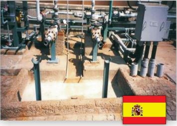
The local ENECON Ibérica Fluid Flow Systems Specialist was contacted to help find a solution to this chemical attack problem. It was recommended that the damaged concrete surfaces first be repaired and rebuilt with
