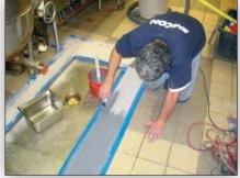
After damaged materials were removed, DuraQuartz was applied to provide a smooth transition from the quarry tile floor to the rim of the trough.
