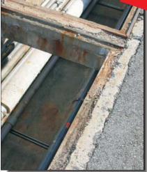
It was suggested that all of the loose material in the damaged areas surrounding the access plates be removed and then cleaned. **ENECRETE DuraQuartz** was then used to build up and level out the damaged concrete surfaces.
