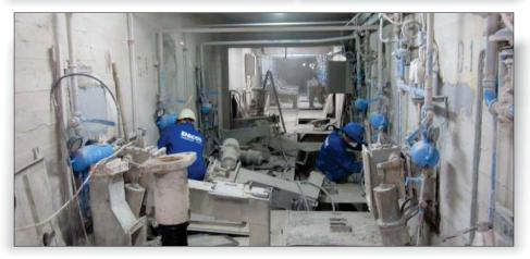
One of the largest cement factories in Turkey was having trouble with leaking silos where raw materials are stored. Two silos carrying a total of 7,000 tons of hot raw material were leaking through worn concrete walls at the silo bases. The engineers at the cement factory have tried a number of different concrete repairs over the years but none of them solved the problem.
