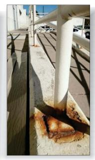
A candy manufacturer in the western United States contacted ENECON in the hope of solving a severe corrosion issue that was not only unsightly but beginning to impact the steel railing's structural integrity.
