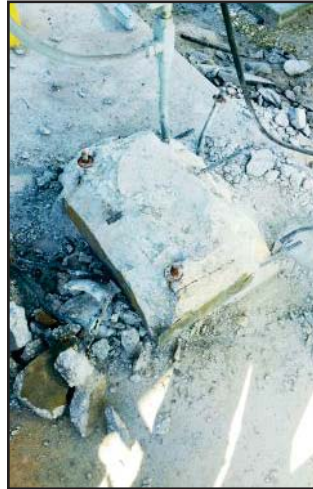
Damaged pump base.
