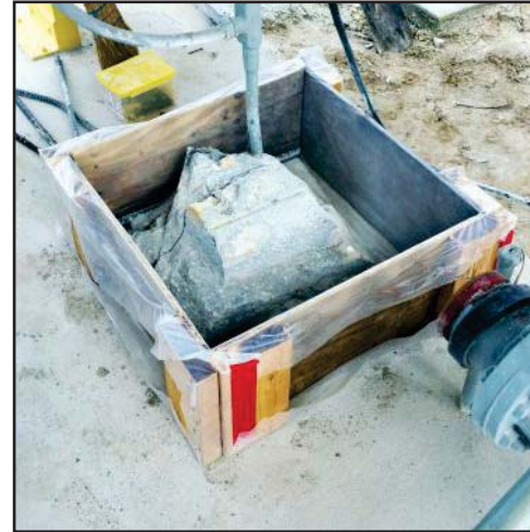
Former with plastic sheeting.
