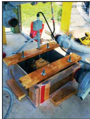
Bolt placement guides.
