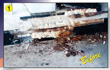
A very popular chain of Pennsylvania gas stations & convenience stores was experiencing severe corrosion and erosion on their gas pump island curbs. It was a potential hazard to customers and employees in addition to being very unsightly.
