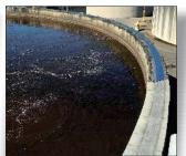
The steel plating on this clarifier tank rim, which serves as a track for the tank's scraping bridge wheels, had been in service for 15 years. Located at a Southern Louisiana wastewater treatment facility, the bridge makes approximately one full rotation every minute.
