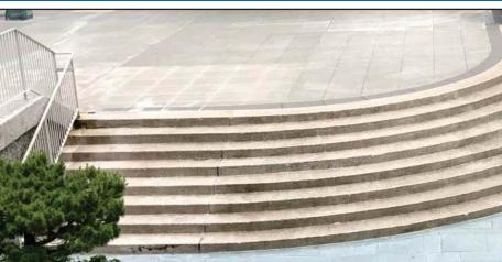
These outdoor courtyard steps in Seattle, WA have heavy foot traffic all day long from general sidewalk use and office building/restaurant loose material. entry ways in the courtyard. Over the past decade. the condition of these steps has deteriorated with cracks and concrete loss.
