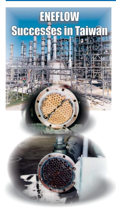
At a chemical fiber (polyester, nylon, etc.) manufacturing plant - one of the largest companies in Taiwan - the oil cooler for a large air compressor was experiencing scaling problems.
