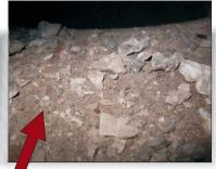
Almost immediately after the *ENEFLOW* was installed, the existing scale began to dissolve and loosen, eventually falling off of the interior surfaces of the boiler and collecting at the bottom where it could be removed by maintenance personnel.
