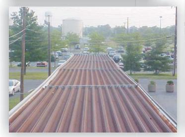
These metal canopy roofs of the passenger terminal at a major US Air Force Base had deteriorated badly because previously applied conventional paint systems provided only limited protection. Jet fumes contributed to the paint system's failure and
