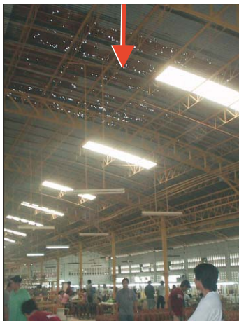
Note the holes in roof.
