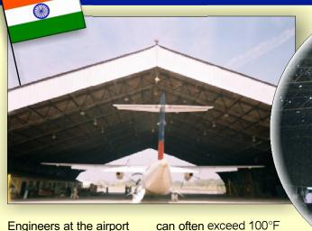
Engineers at the airport in Calcutta were tired of "seeing stars" through the roof of some of their airplane hangars. Conventional tar-felting could not provide the long-term repair solution they were looking for on these corrugated metal roofs. Each hangar is over 32,000 square feet.
