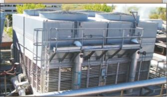
At this major pharmaceutical plant located in Pennsylvania, these 5 cooling towers sit atop I-beam supported grated platforms. These I-beams had been suffering for years from corrosion caused by atmospheric pollution mixing with the water splashing from the large cooling towers. The tight spacing of the grated metal supports also trap moisture and accelerate the corrosion problems.
