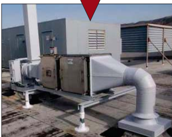
Rooftop ventilation filter station. Prepared by pressure washing the entire surface then two coats of ENESEAL® CR were applied to prevent against future corrosion.
