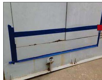
Electrical cabinet. Prepared by pressure washing then two coats of ENESEAL® CR.
