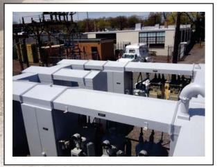
A mid-Atlantic power company is partnering with ENECON Corporation to provide a cost effective solution to leaking switchgear cabinets. Many of these cabinets are 70-80 years old and leaks can cause the electrical equipment inside to explode, leading to power outages that can last months.
