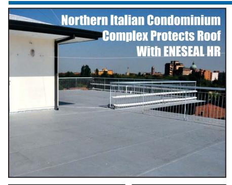
The conventional tar paper and aluminum coated roof of this condominium complex in northern Italy needed to be resurfaced. The government enacted regulations on aluminum coated roofs near airports due to reflectiveness and their effect on the providing heat planes passing overhead. The aluminum coating was also failing in many areas.
