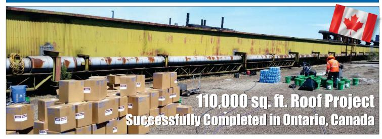
This factory roof in Ontario, Canada, was experiencing leaks, big and small, through their 40+ year old roof. This is a built up roof or "BUR", which is tar & gravel on top of insulation laying on corrugated sheet metal. There are over 20 million square feet of roofs at this facility!
