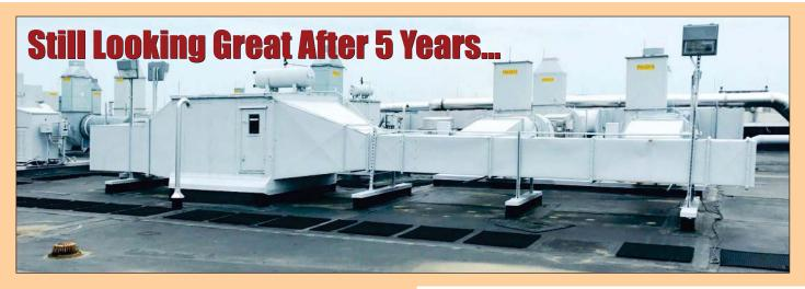
After 5 years since initial protection with ENESEAL CR, these rooftop air handler fans, pads and ductwork continue to be protected from environmental corrosion.
