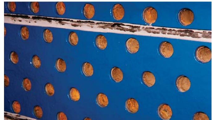
CeramAlloy CL+ applied to complete the project.
