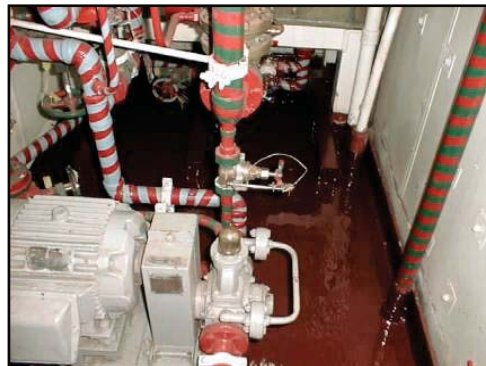
First coat of CeramAlloy Grey color followed by a second coat of CeramAlloy AFFF Red
