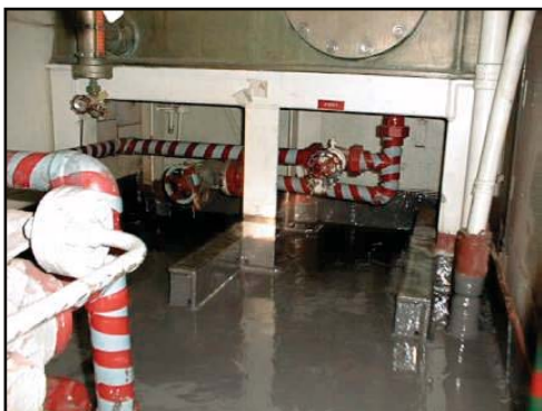
First coat of CeramAlloy Grey color followed by a second coat of CeramAlloy AFFF Red
