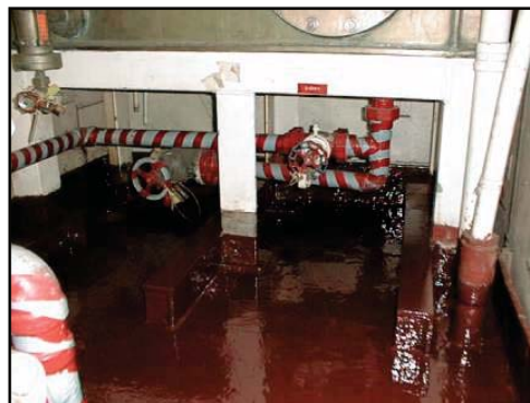
First coat of CeramAlloy Grey color followed by a second coat of CeramAlloy AFFF Red
