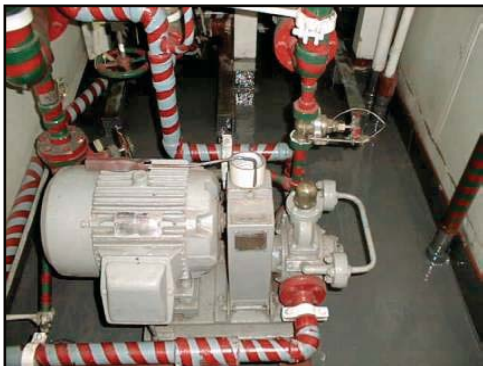
First coat of CeramAlloy Grey color followed by a second coat of CeramAlloy AFFF Red
