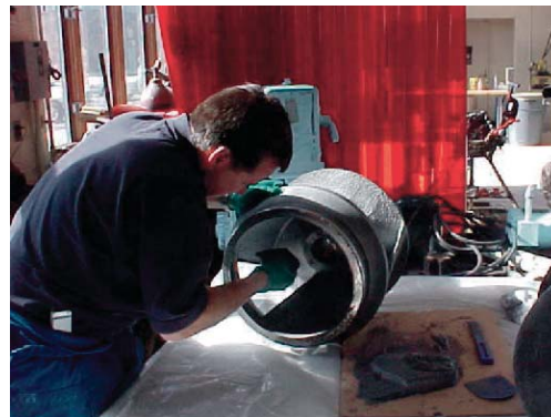
CeramAlloy CP + AC was used to smooth out and rebuild eroded areas of both impellers.
