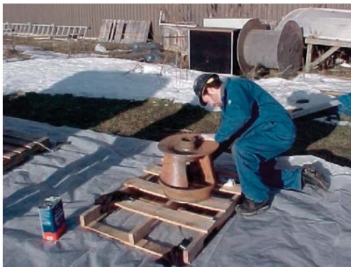
Impellers placed on pallets outdoors and then grit blasted to minimum 3 mil profile.
