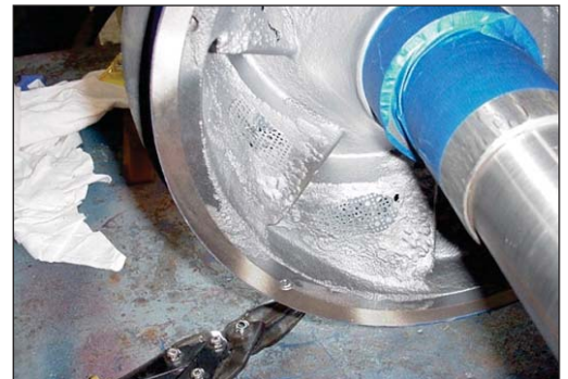
Reinforcing 'mesh' and DurAlloy applied over holes
