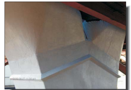
DurAlloy applied over entire extractor shell.
