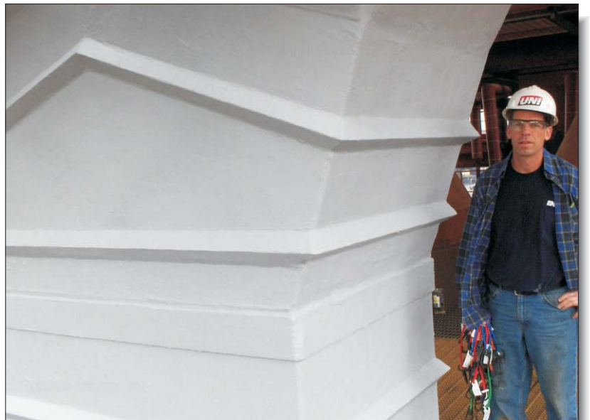
After totally encapsulating the unit in DurAlloy, ENESEAL CR was used to provide optimum corrosion resistance and a uniform look.
