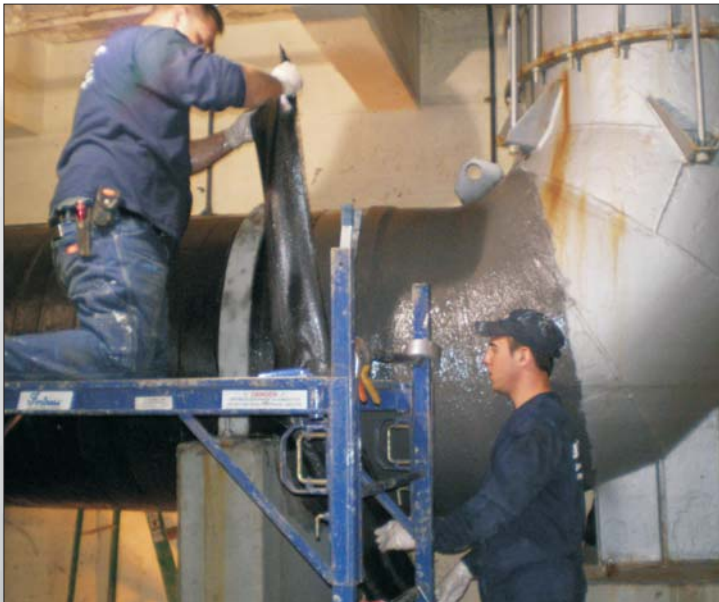
DuraWrap Carbon Fiber, impregnated with DuraWrap Polymers, being wrapped around pipe section.
