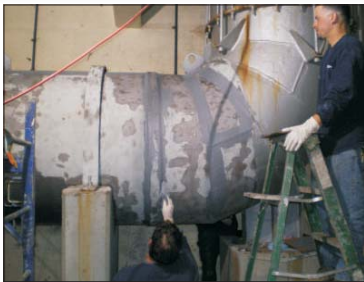
After grit blasting, leaks repaired with DurAlloy.
