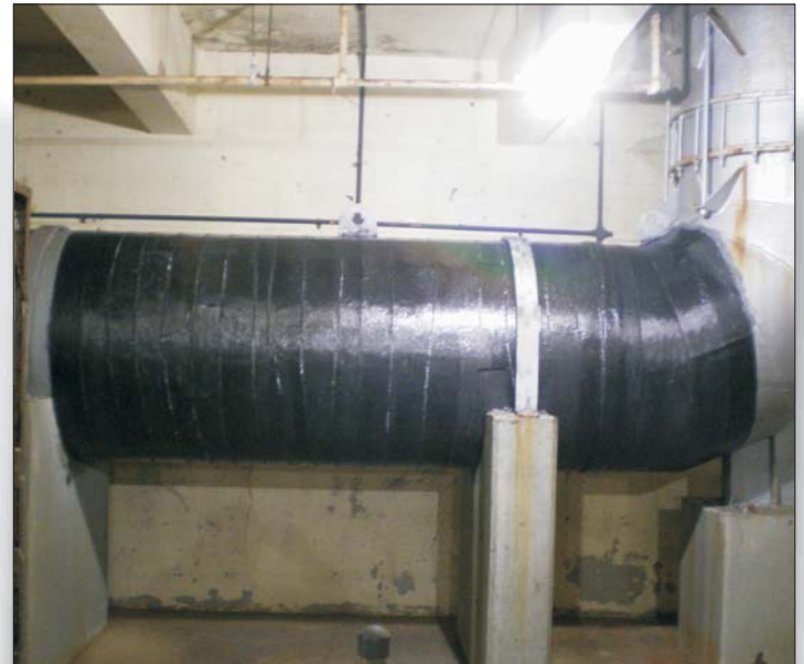
Completed DuraWrap System.
