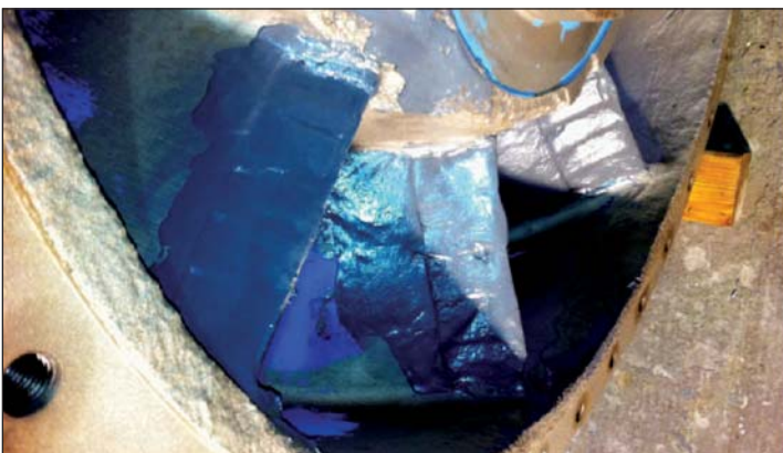
CeramAlloy CP+AC used to rebuild the vanes to their original size.
